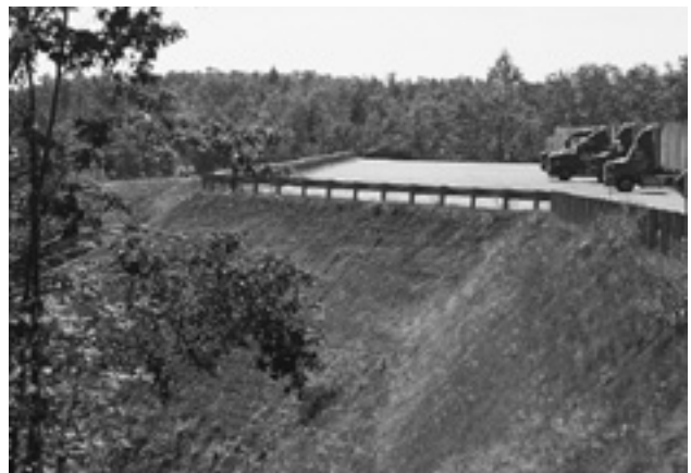
Completed Sierra® Slope at a plant expansion facility.
