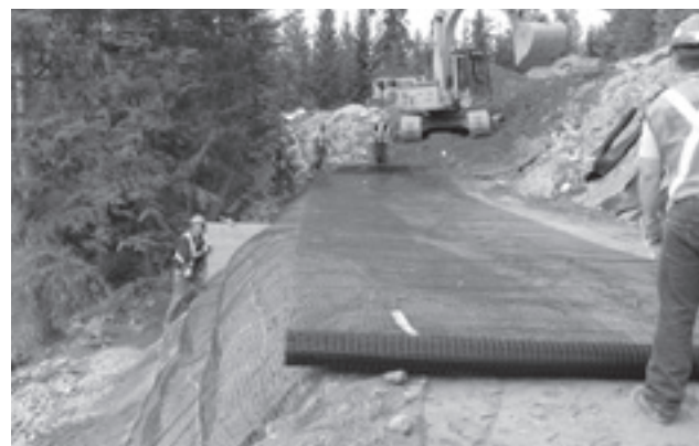
Tensar BX Geogrids used for secondary reinforcement are typically rolled out parallel to the slope face.
