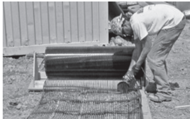
Field cutting the UX Geogrid.
