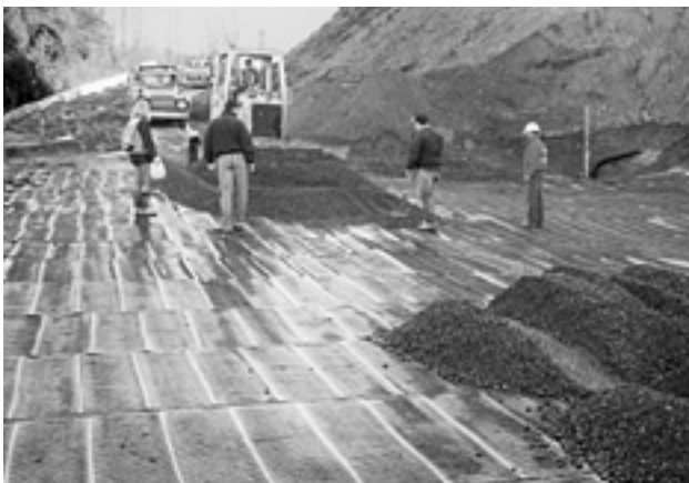
UX Geogrid and fill placement.
