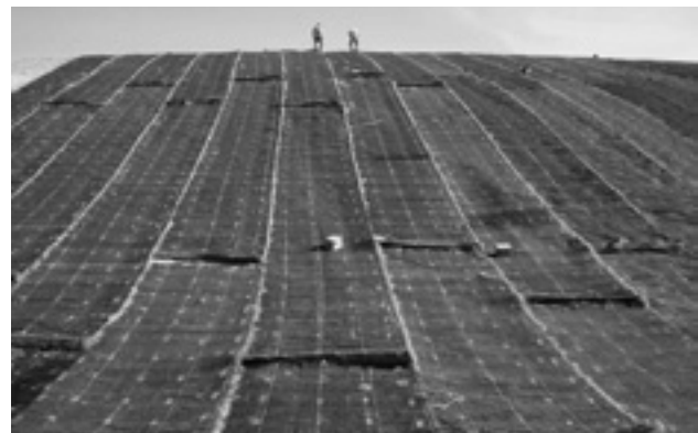
RECP installation down the face of the slope.
