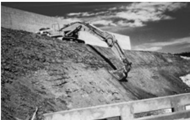
Slope face is graded smooth in preparation for RECP installation.
