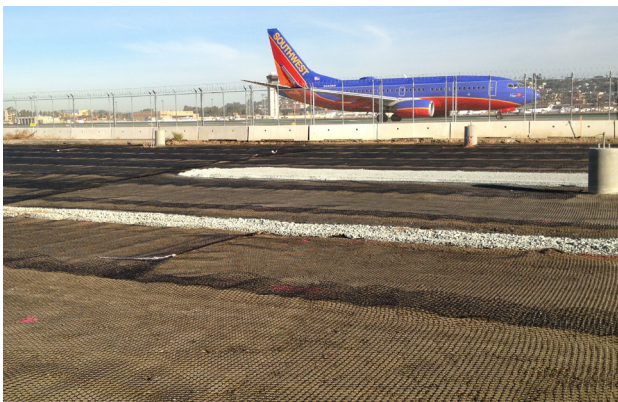
Tensor® TriAx® Geogrid allowed for an optimized pavement section to reduce the aggregate base layer by 45% while providing superior base confinement.
