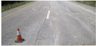
During the 2018 site visit, additional cracking was observed in the unreinforced section.
