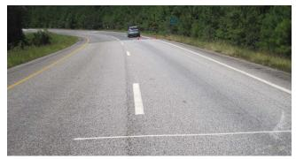
The GlasGrid reinforced section was also evaluated in 2018. After 60 million ESALs, cracking was starting to appear but limited to the 18 yr. old construction joint.
