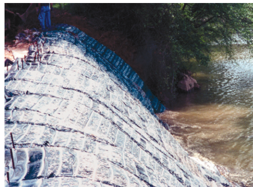
Triton Mattresses now protect the riverbank from erosion.
