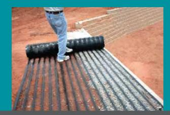
Rolling Grid Parallel to Wall Face = Fewer Cuts = Faster Install
